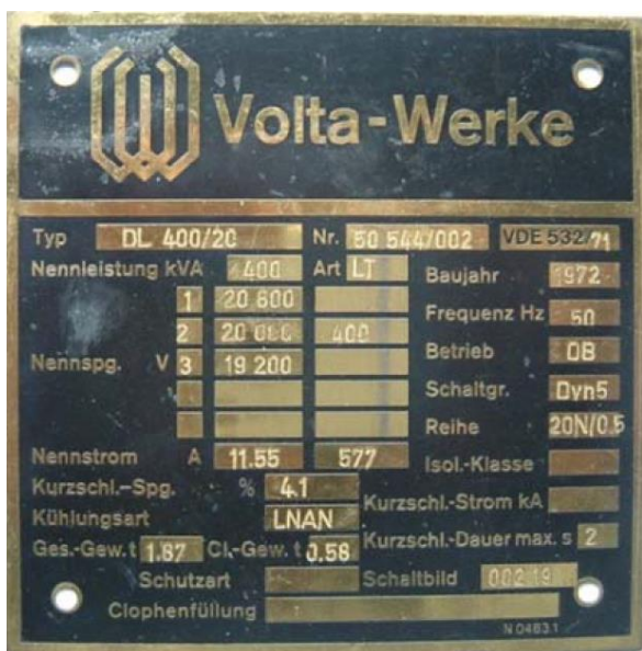
Figure 3: Name plates from transformers: left = containing PCB (Kühlungsart LNaN) and right – not containing PCB (cooling = ONAN)
