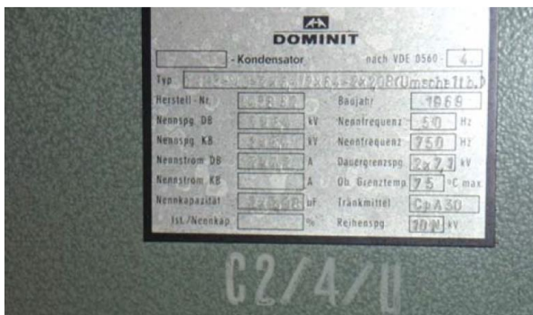
Figure 4: Example for name plates from capacitors. Left: Tränkmittel (= liquid) CpA 30 refers to Clophen A30 (source (Müller, 2011); right: ‘Pyranol’ refers to commercial PCB product (source (UNEP, 2010)
